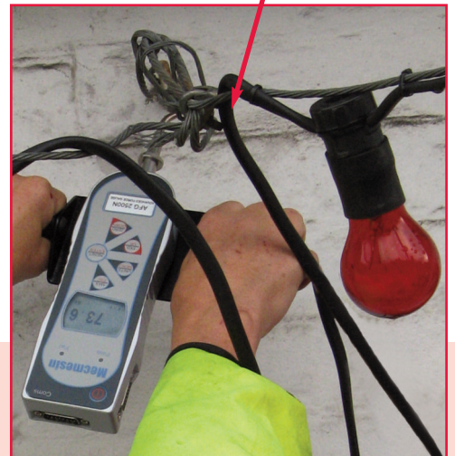
Eyebolt securing the Christmas lights to the building
